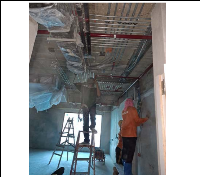
Activity Installation Pipe Sprinkler Area Mock up Room No.24 Floor 8 Date : 7 September 2563
