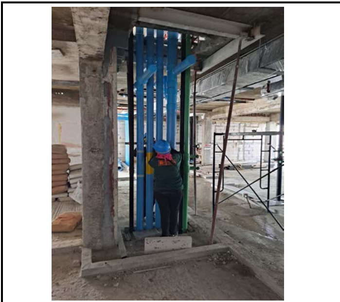
Activity HWR,HWS Pipe Insulation in Shaft Area . Floor 13-16 Date : 7 September 2563
