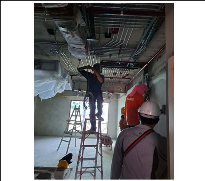
Activity Installation Pipe Sprinkler Area Mock up Room No.24 Floor 8 Date : 7 September 2563
