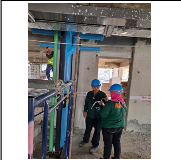
Activity Installation CW,HW Pipe Floor 16 Date : 7 September 2563
