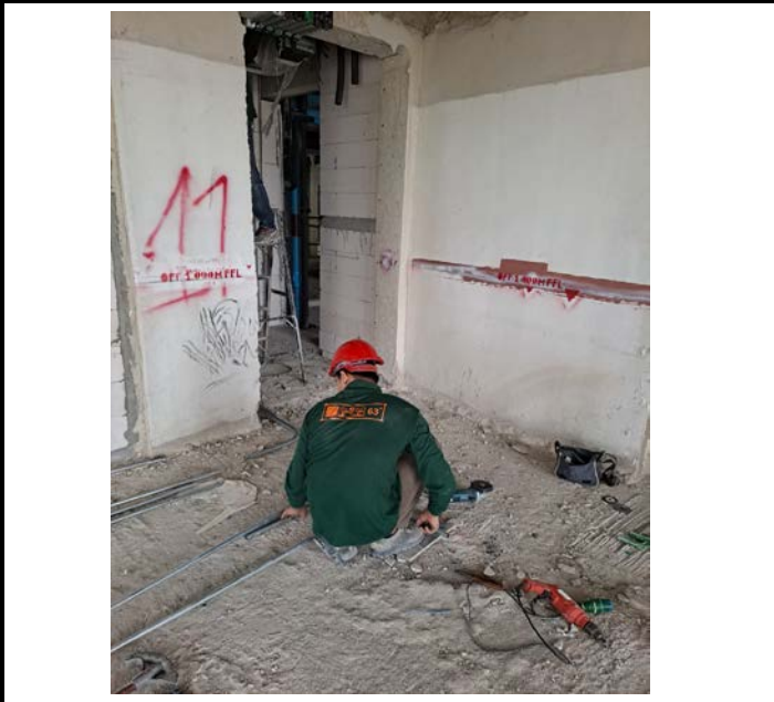
Activity Installation of Electrical Pipe Above the ceiling for the Room. Floor 14 Date : 7 September 2563
