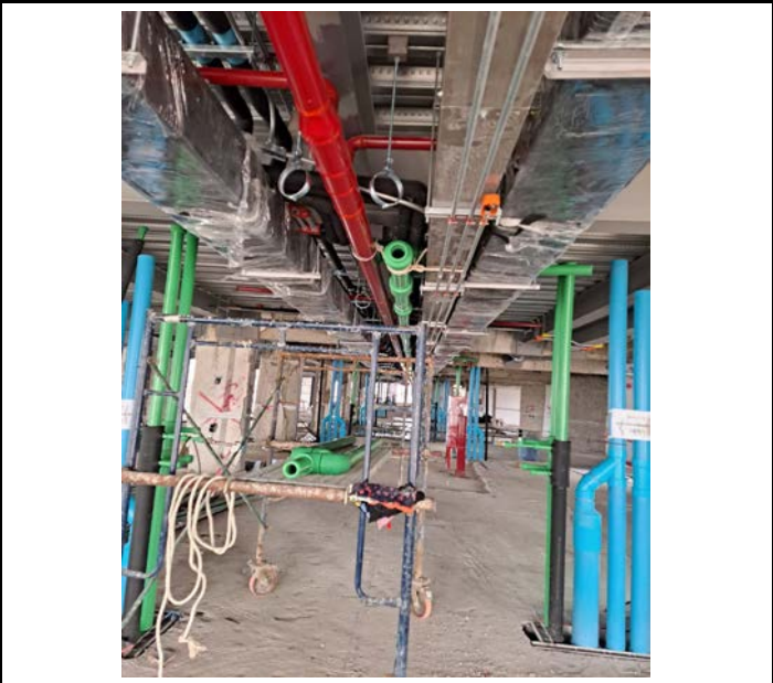
Activity Installation CW,HW Pipe Area Corridor Floor 16 Date : 8 September 2563
