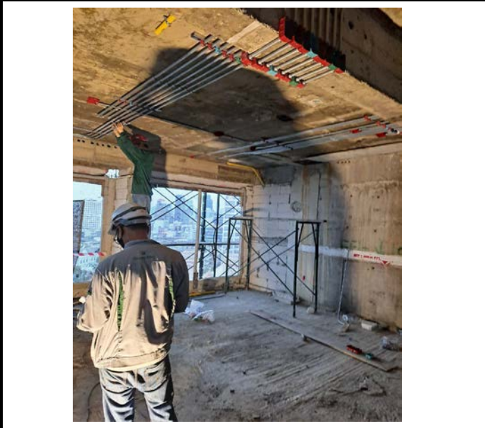
Activity Installation of Electrical Pipe Above the ceiling for the Room. Floor 14 Date : 10 September 2563
