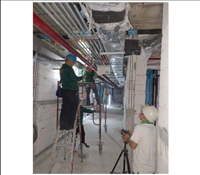
Activity Installation CW,HW Pipe Area Corridor. Floor 12 Date : 11 September 2563
