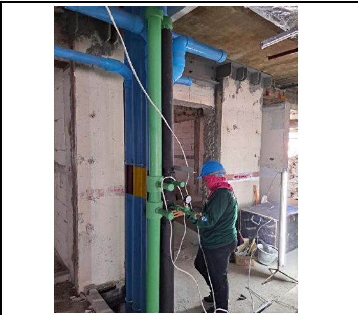
Activity Installation the Pipe Holder Floor 6-16 Date : 11 September 2563
