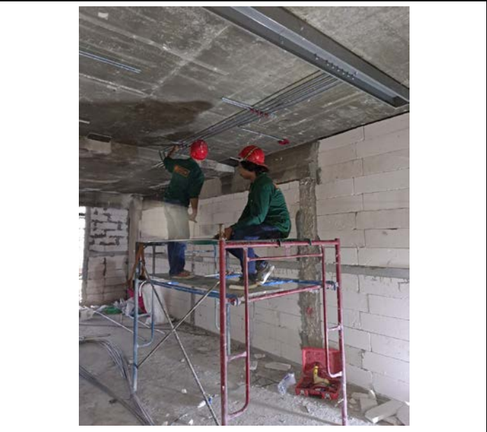
Activity Installation of Electrical Pipe Above the ceiling for the Room. Floor 13 Date : 11 September 2563
