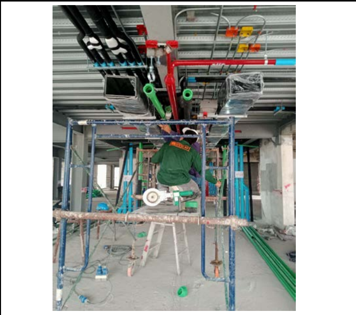
Activity Installation CW,HW Pipe Area Corridor. Floor 16 Date : 13 September 2563
