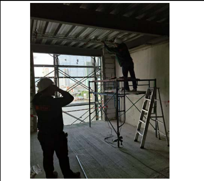
Activity Installation of Electrical Pipe Above the ceiling for the Room. Floor 13 Date : 14 September 2563
