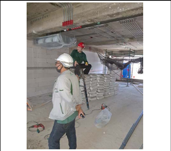
Activity Installation of Electrical Pipe Above the ceiling for the Room. Floor 08 Date : 16 September 2563
