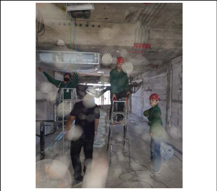
Activity Installation of Electrical Pipe Above the ceiling for the Room. Floor 08 Date : 16 September 2563
