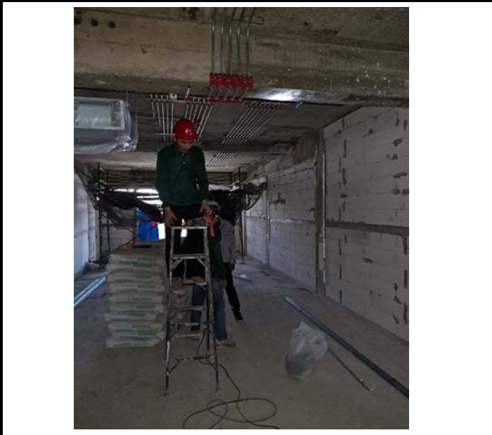
Activity Installation of Electrical Pipe Above the ceiling for the Room. Floor 08 Date : 16 September 2563
