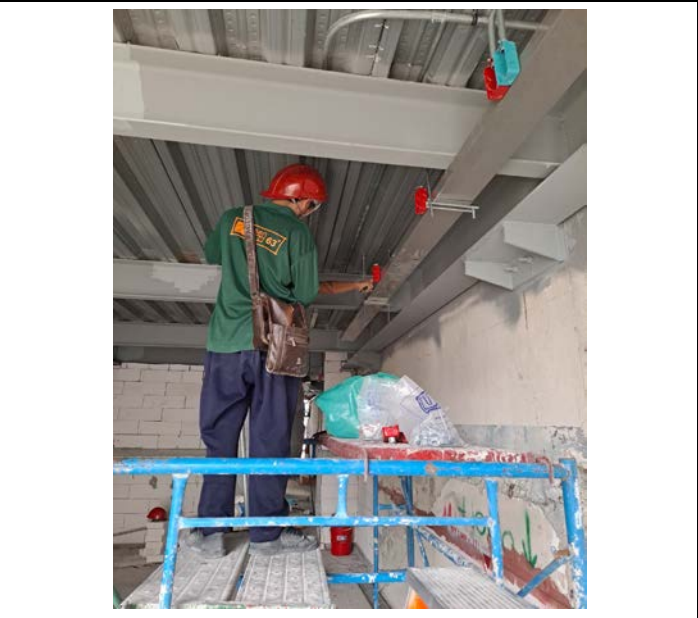
Activity Installation of Electrical Pipe Above the ceiling for the Room. Floor 13 Date : 17 September 2563
