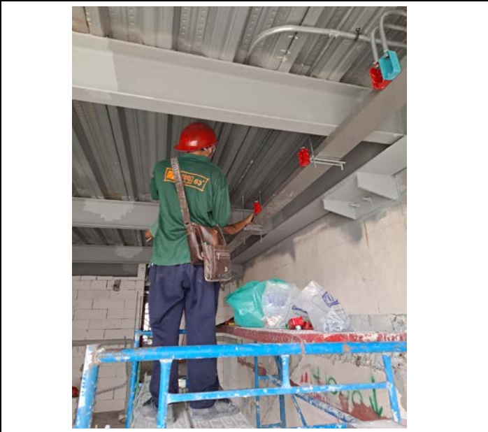
Activity Installation of Electrical Pipe Above the ceiling for the Room. Floor 13 Date : 17 September 2563
