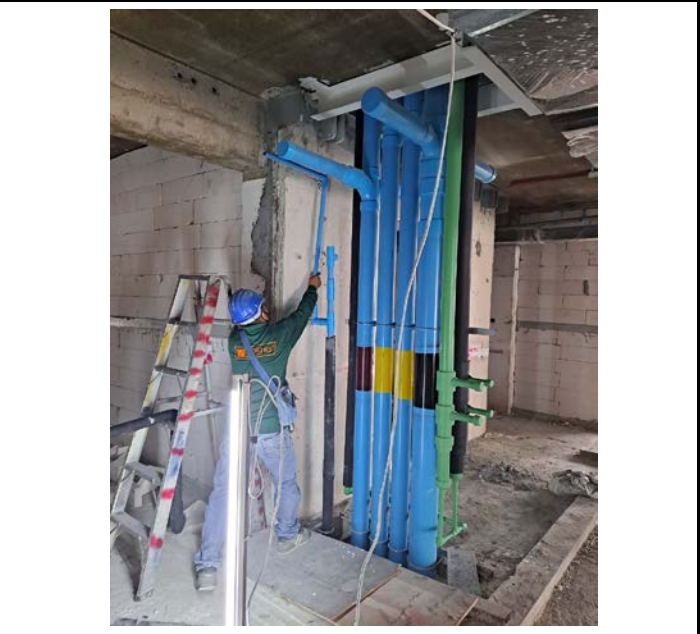
Activity Installation The Shaft Area Drain Floor 6-15 Date : 17 September 2563
