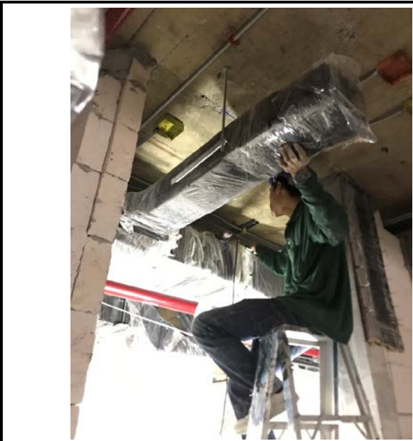
Activity Installation of Duct In The Room Floor 10 Date : 18 September 2563
