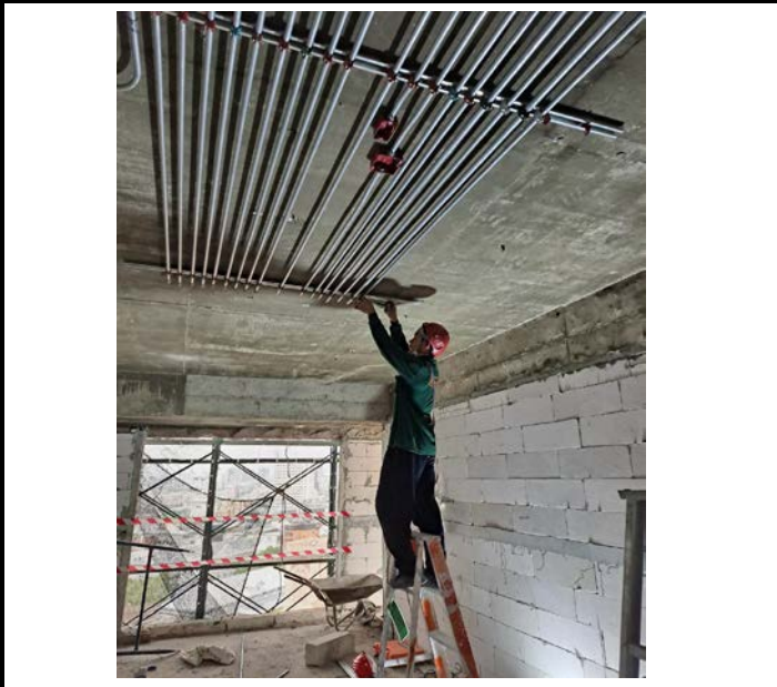
Activity Installation of Electrical Pipe Above the ceiling for the Room. Floor 13 Date : 18 September 2563
