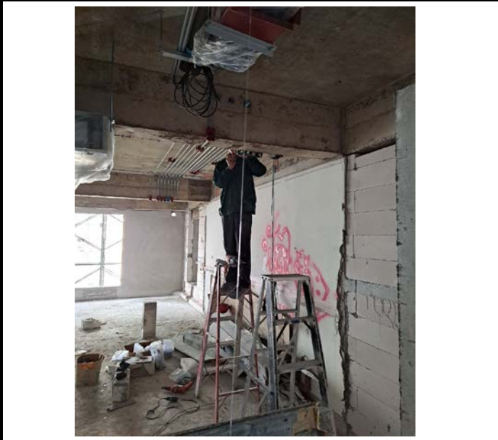
Activity Installation of Electrical Pipe Above the ceiling for the Room. Floor 08 Date : 21 September 2563
