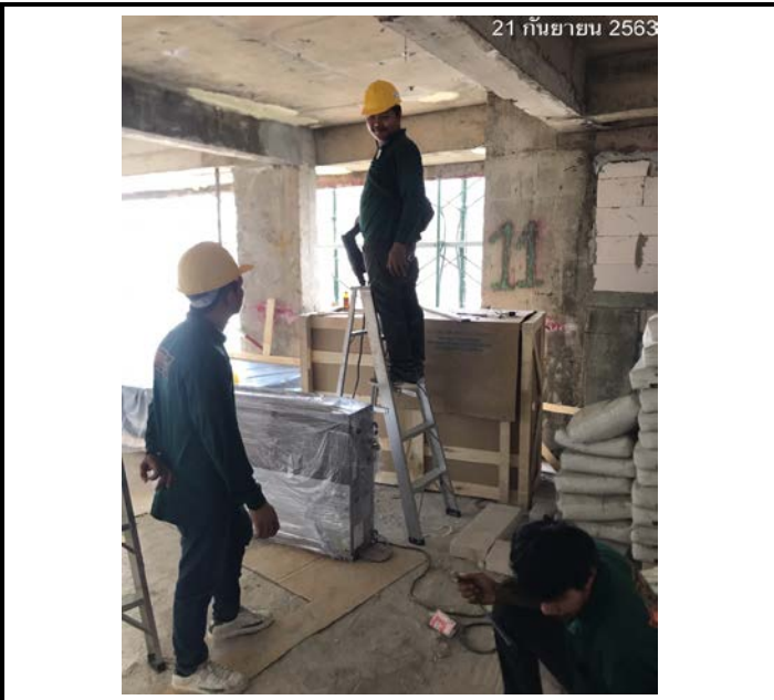
Activity Installation of Air Conditioner Floor 11 Date : 21 September 2563
