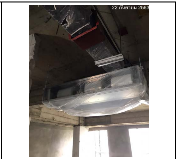
Activity Installation of Air Conditioner Floor 09 Date : 22 September 2563
