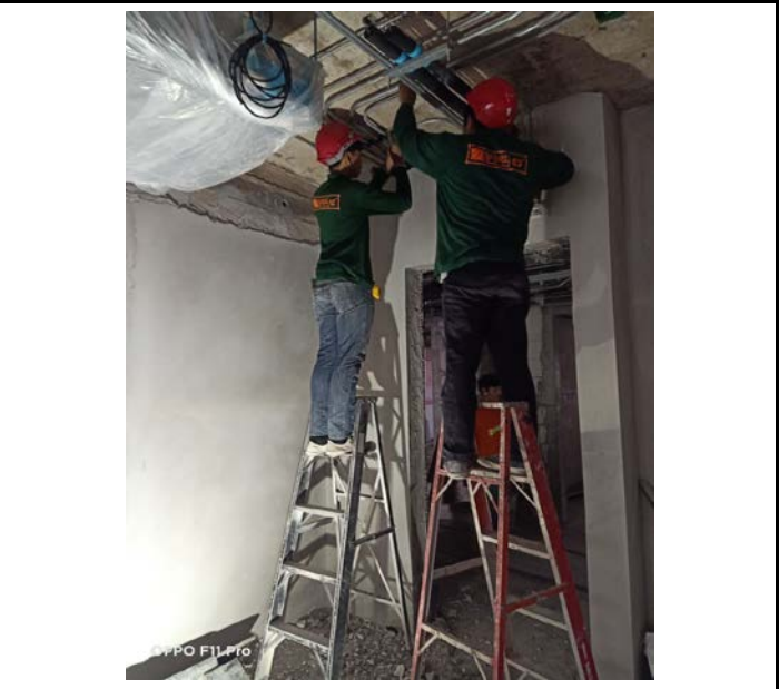
Activity Installation of Electrical Pipe Above the ceiling for the Room. Floor 08 Date : 22 September 2563
