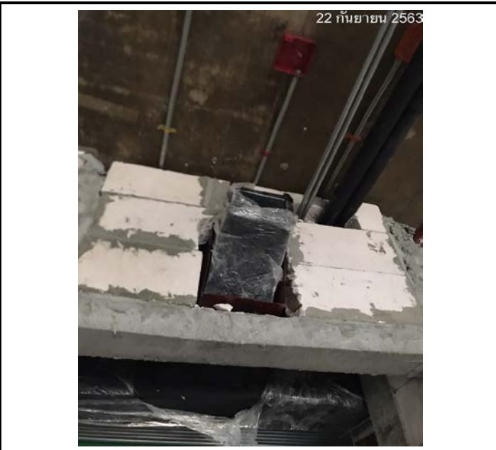
Activity Installation of Duct In The Room Floor 12 Date : 22 September 2563
