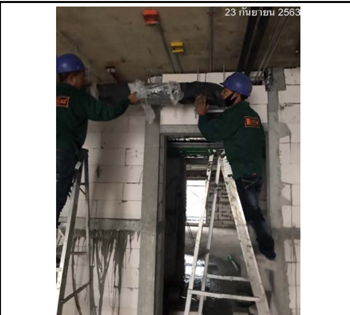
Activity Installation of Duct In The Room Floor 15 Date : 23 September 2563
