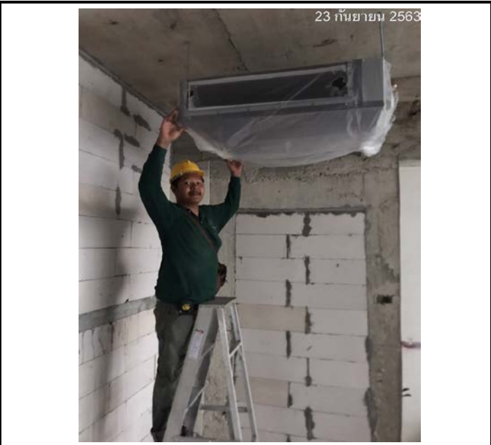
Activity Installation of Air Conditioner Floor 11 Date : 23 September 2563
