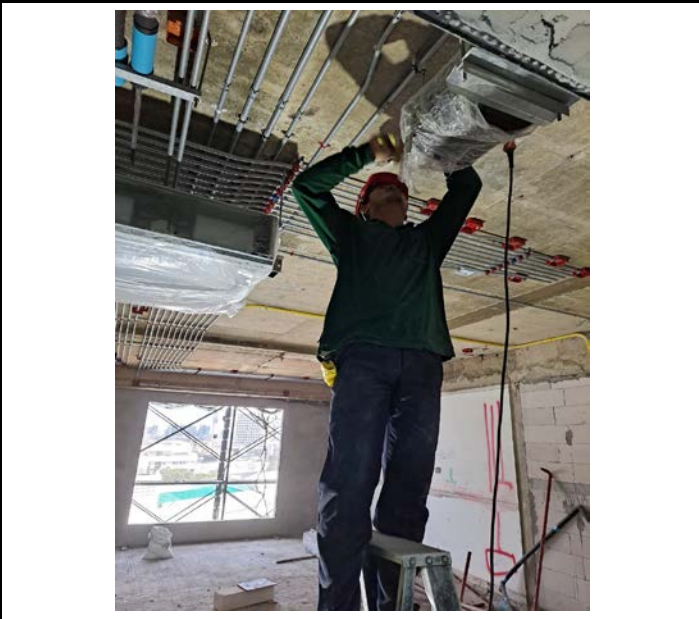
Activity Installation of Electrical Pipe Above the ceiling for the Room. Floor 08 Date : 24 September 2563
