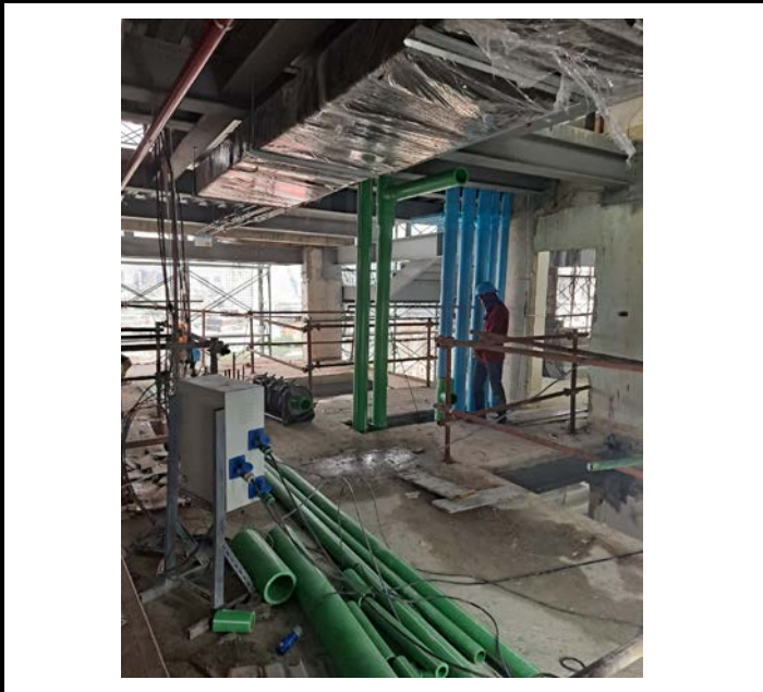
Activity Installation CW,HW Pipe For Shaft Floor 12 Date : 24 September 2563
