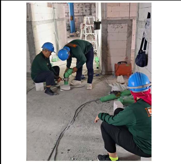
Activity Installation CW,HW Pipe For Corridor Floor 12 Date : 24 September 2563
