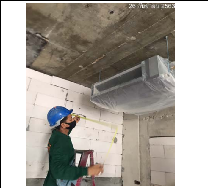
Activity Inspect The Distance Of The Air Conditioner Floor 09 Date : 26 September 2563
