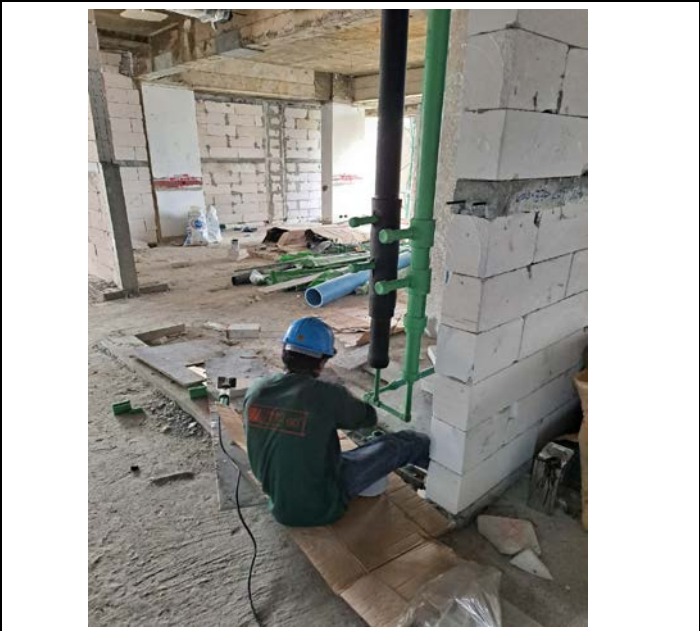
Activity Installation CW,HW Pipe For Shaft Floor 05 Date : 26 September 2563
