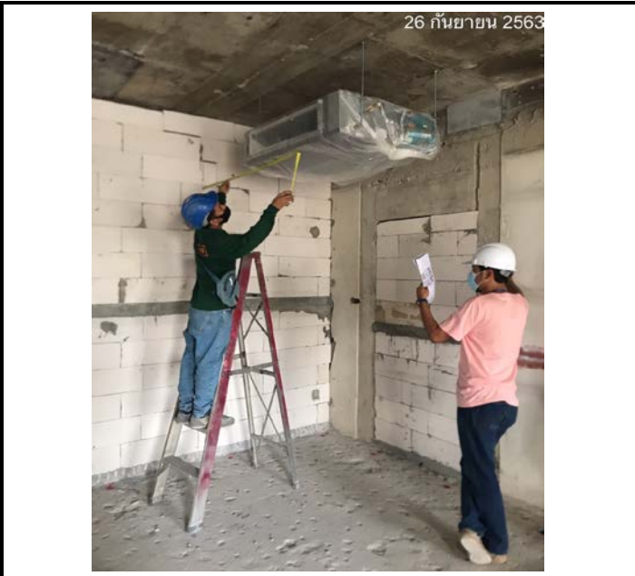
Activity Inspect The Distance Of The Air Conditioner Floor 09 Date : 26 September 2563
