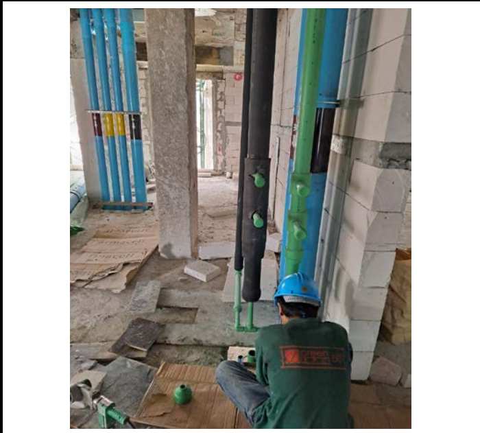
Activity Installation CW,HW Pipe For Shaft Floor 05 Date : 26 September 2563
