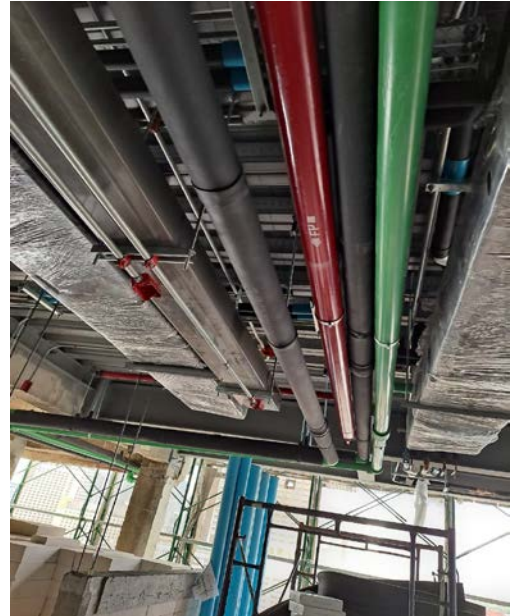
Activity Inspect The Installation Of Hot Water, Cold Water Pipes Floor 16 Date : 29 September 2563
