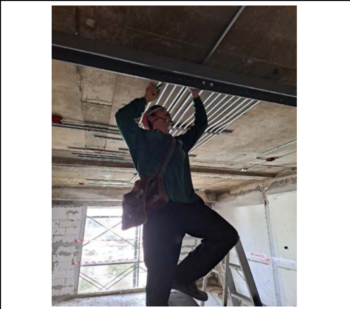
Activity Installation of Electrical Pipe Above the ceiling for the Room. Floor 10 Date : 29 September 2563
