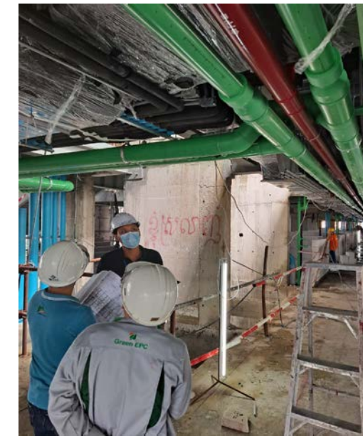
Activity Inspect The Installation Of Hot Water, Cold Water Pipes Floor 16 Date : 29 September 2563
