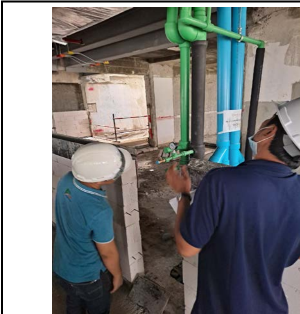
Activity Inspect The Installation Of Hot Water, Cold Water Pipes Floor 16 Date : 29 September 2563
