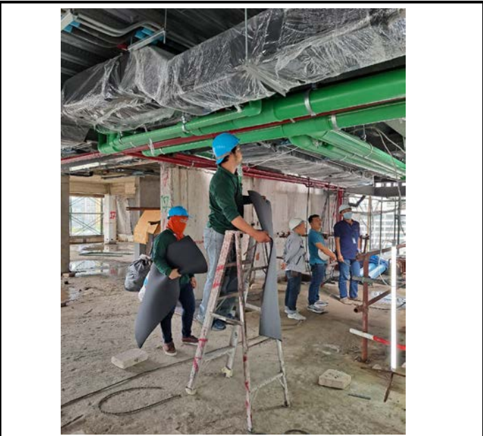
Activity Insulated Cold And Hot Water Pipes At the Corridor Floor 16 Date : 29 September 2563
