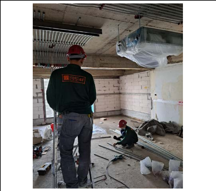
Activity Installation of Electrical Pipe Above the ceiling for the Room. Floor 11 Date : 30 September 2563
